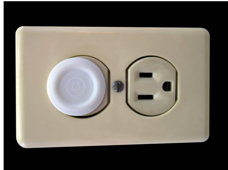
Insert plastic safety plugs in unused electrical outlets
